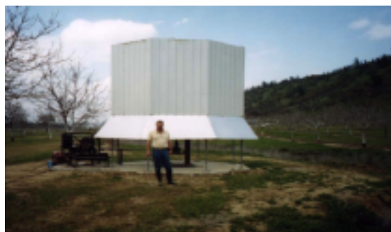
Photo. 1 - SIS installed in California – USA (2000)
